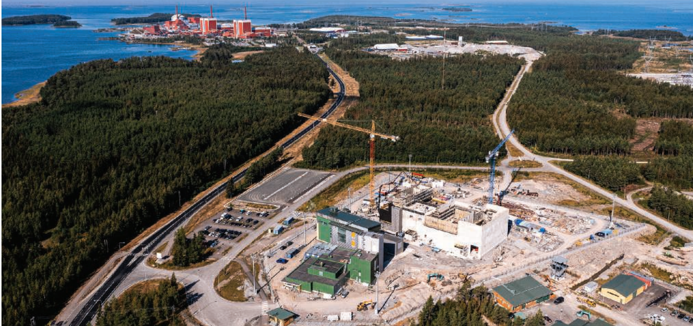
Onkalo's encapsulation plant (white) sits atop an ant's nest of underground tunnels in this August 2021 photo. Olkiluoto's nuclear power plants can be seen in the distance.
