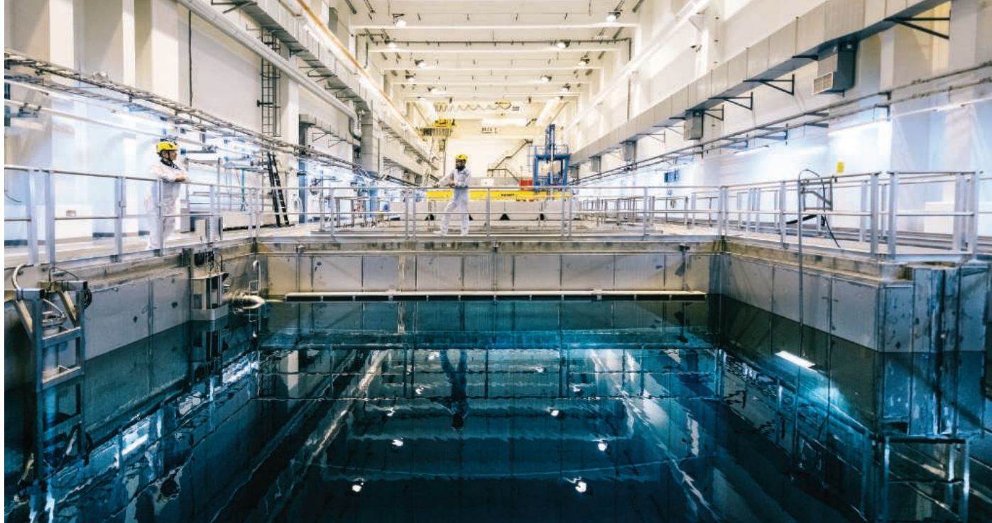
Spent fuel rods from Olkiluoto's nuclear power plants will cool off for several decades in interim storage pools before final burial at Onkalo.
